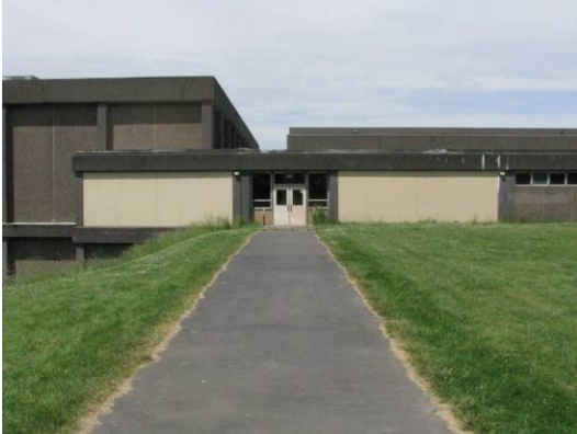
Main building, south elevation, showing blank walls to receive two addition building units (never built) (174A).
